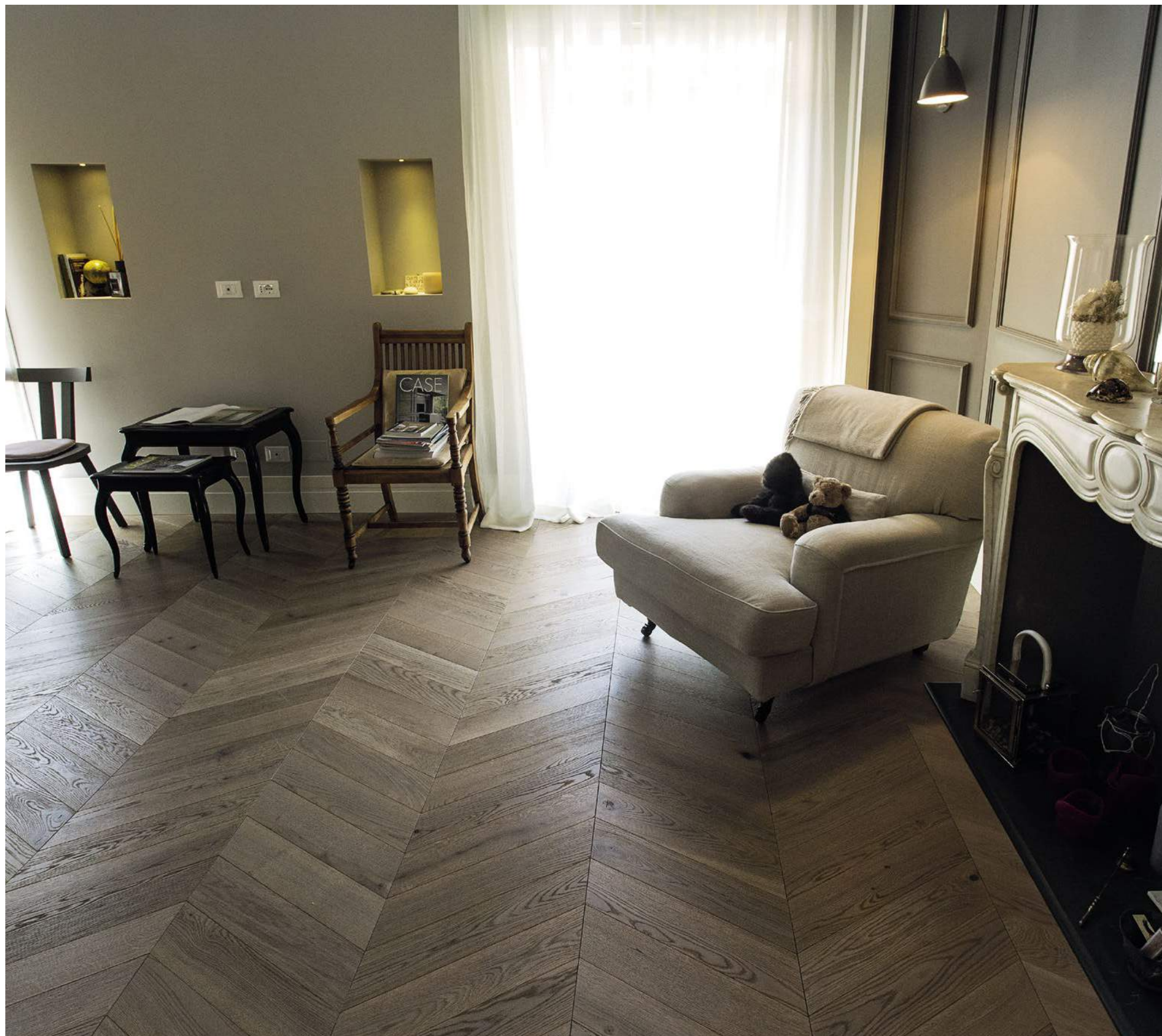
Rovere Nocciola spazzolato e verniciato in scelta natura posato a spina ungherese Oak Nocciola brushed and varnished natura selection hungarian herring bone installation
